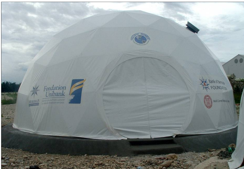
Fig. 11. One of the 30-foot domes completed, Day 5.
