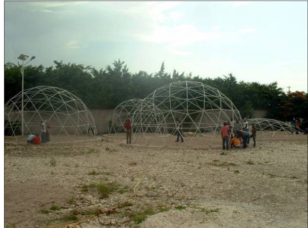
Fig. 4. Progressing with four domes, Day 1.
