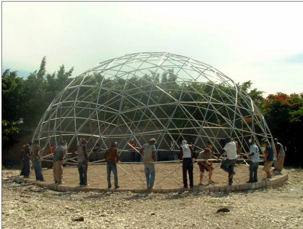
Fig. 5. Lifting a 44-foot dome, Day 1.
