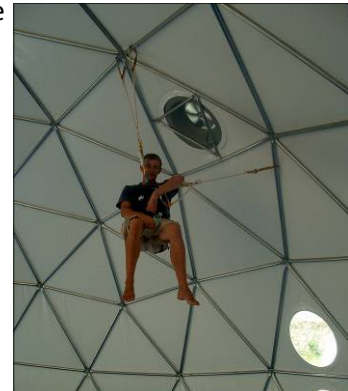
Fig. 10. Installing solar-powered exhaust fans, Day 5.
