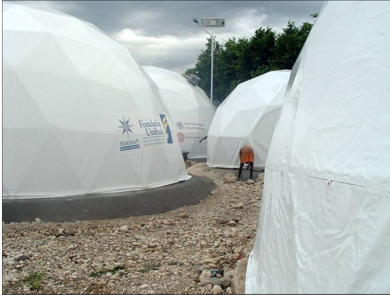
Fig. 12. Finishing the bases and anchoring the domes. Day 5.
