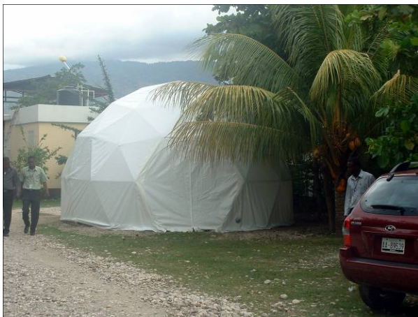
Fig. 13. The second 20-foot dome completed, Day 5.
