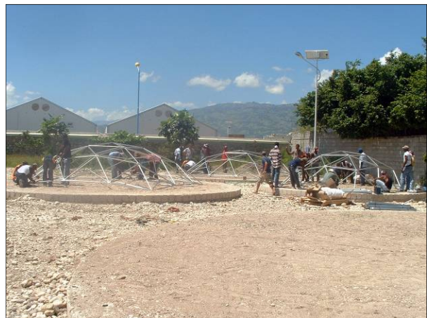
Fig. 3. Starting the Build, Day 1.
